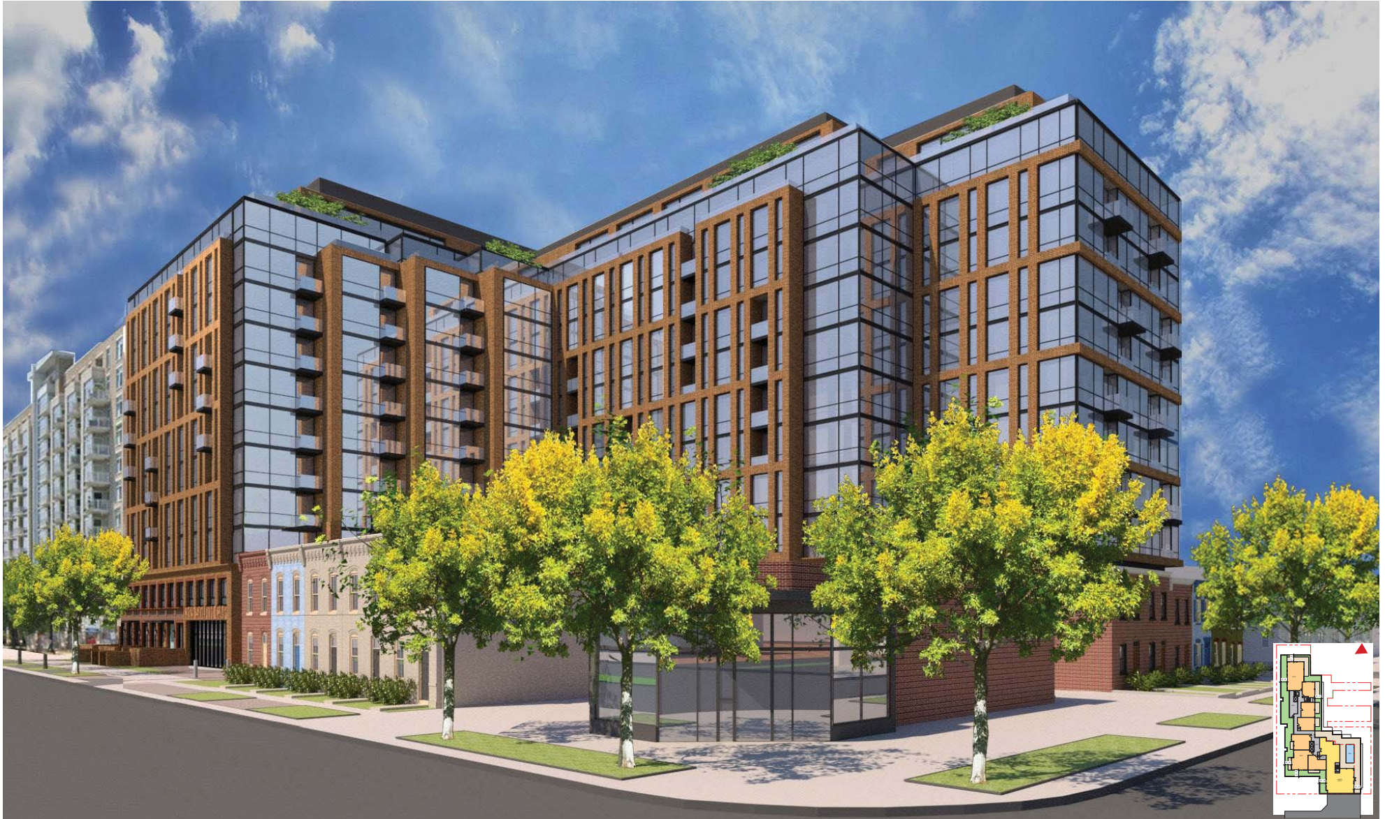
SOME PROPOSED STREET TREES HAVE BEEN REMOVED FOR ILLUSTRATION. SEE PAGE 23 FOR GLASS BALCONY DETAIL.
